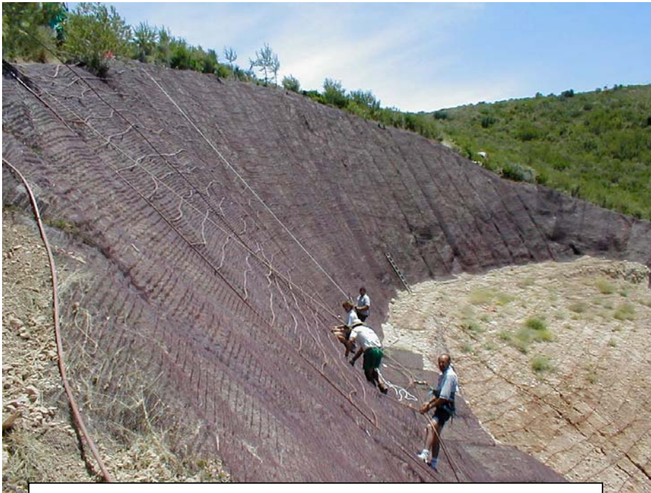
3. Fixing the mesh and the watering lines
